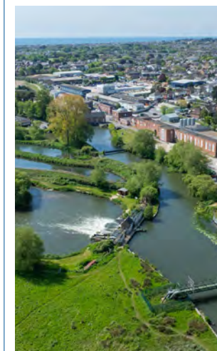
① Knapp Mill Water Treatment Works, Bournemouth Water
