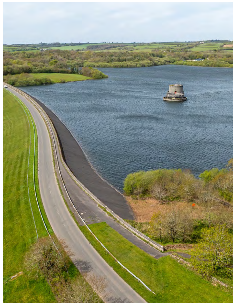
① Roadford reservoir
