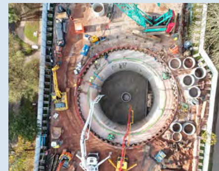
Dawlish wastewater solution
