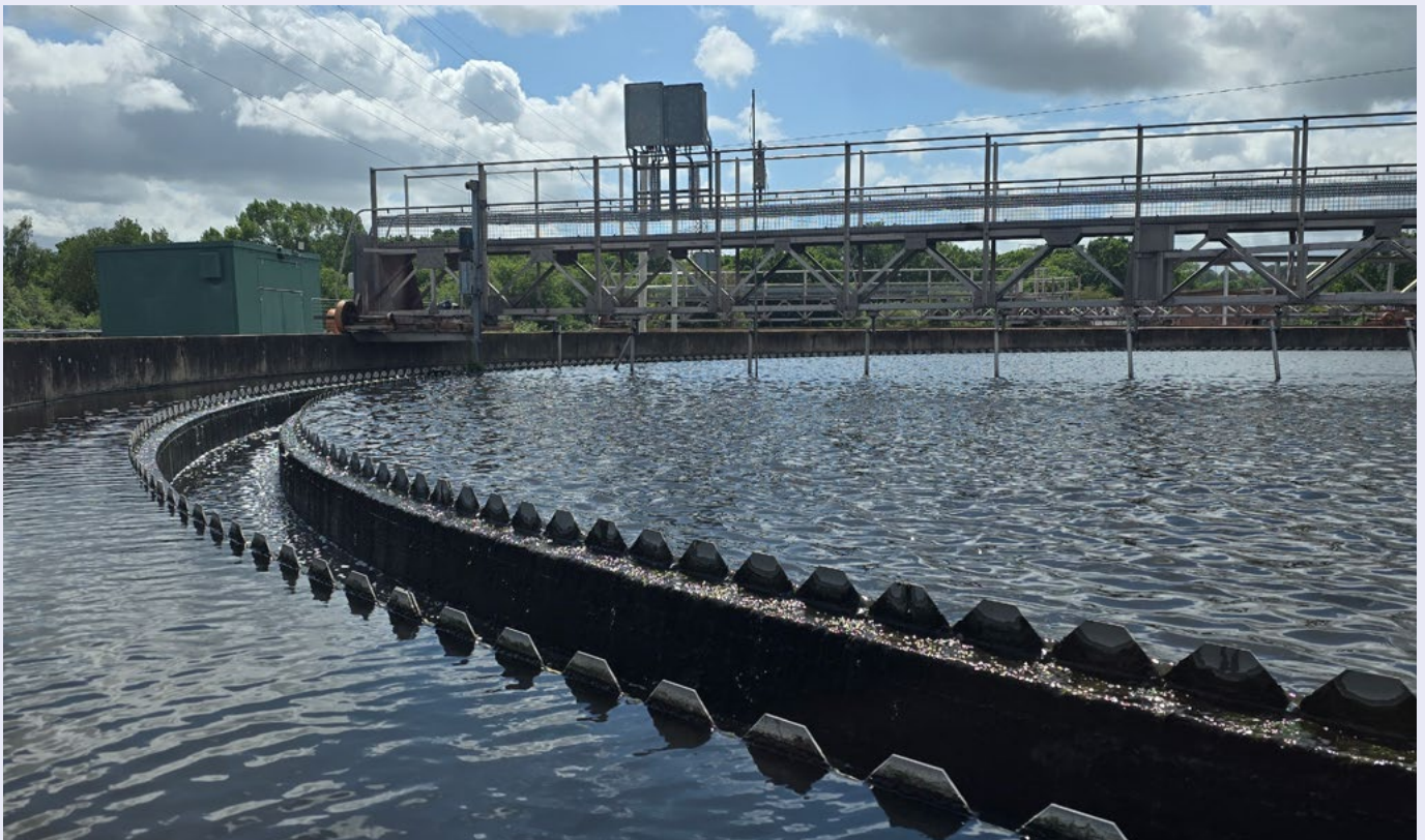
Countess Wear Wastewater Treatment Works, Exeter, is South West Water's largest sewage treatment facility
