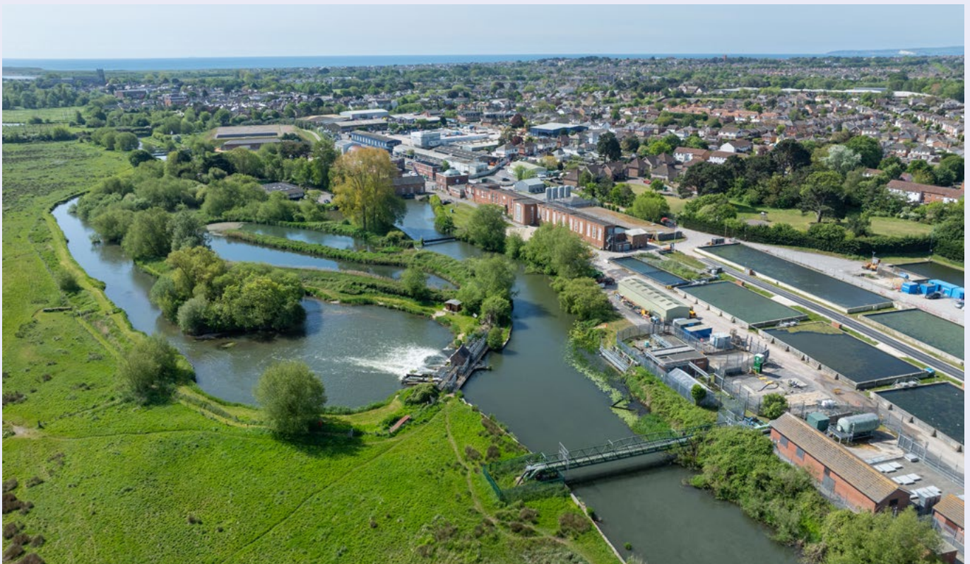
Knapp Mill Water Treatment Works, Christchurch, supplies drinking water to around 163,000 customers across Bournemouth Water's area, including Christchurch, Ringwood, New Milton, Lymington and parts of the New Forest
