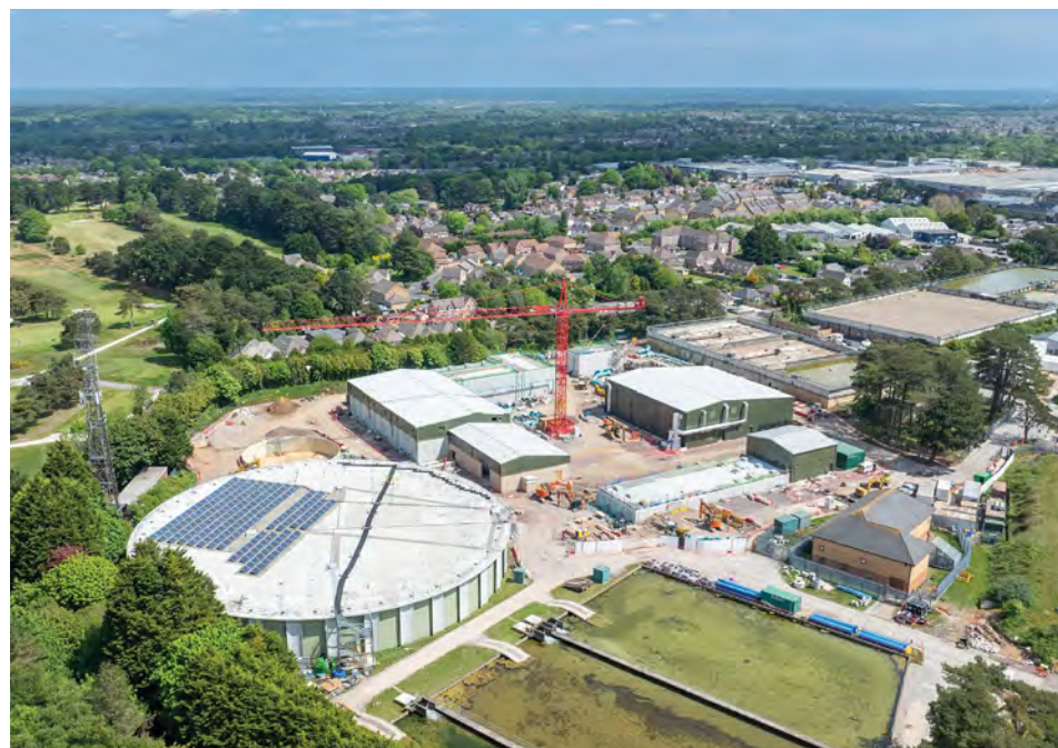
Alderney build in progress
