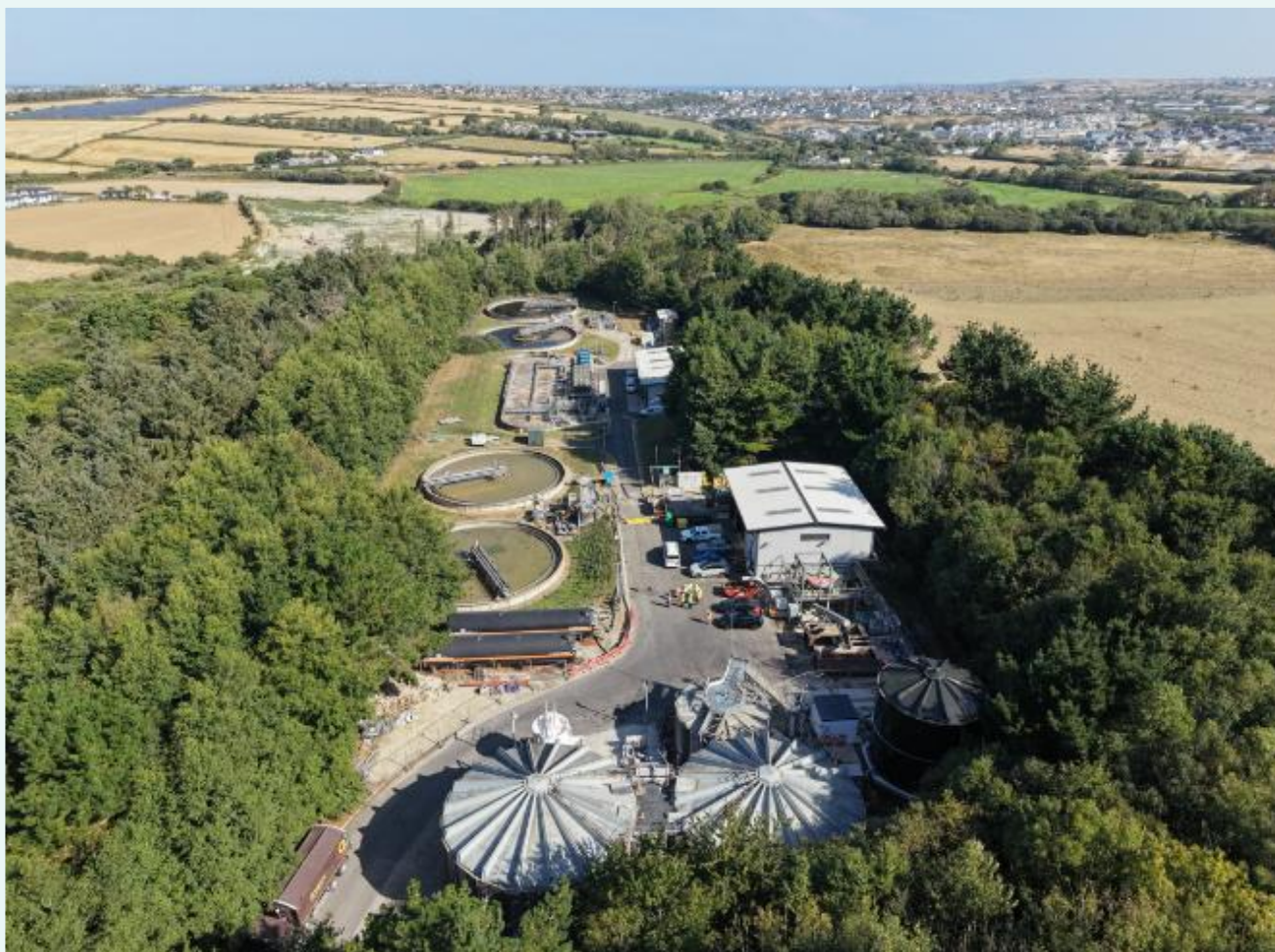
Newquay Wastewater Treatment Works
