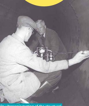
1950s ultrasonic testing of the structural integrity of the Winford tubes
