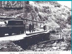
The 1960s saw a range of extreme weather, including flooding in Cheddar Gorge and in the Chew Valley that washed away many bridges and water mains. Temporary diversion pipes were laid to restore supplies.
