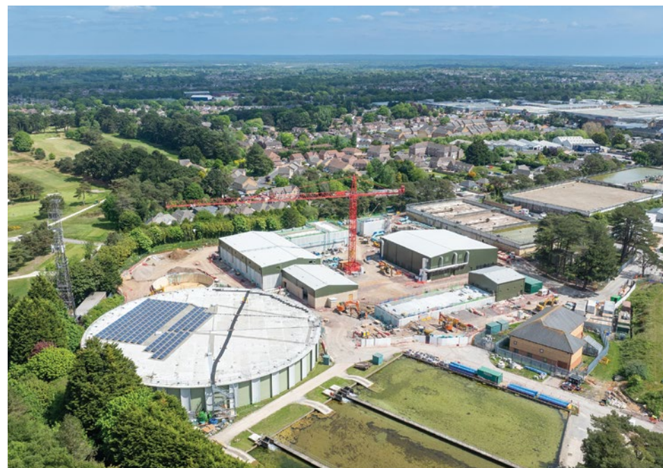
📍 Alderney build in progress
