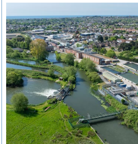
① Knapp Mill Water Treatment Works, Bournemouth Water
