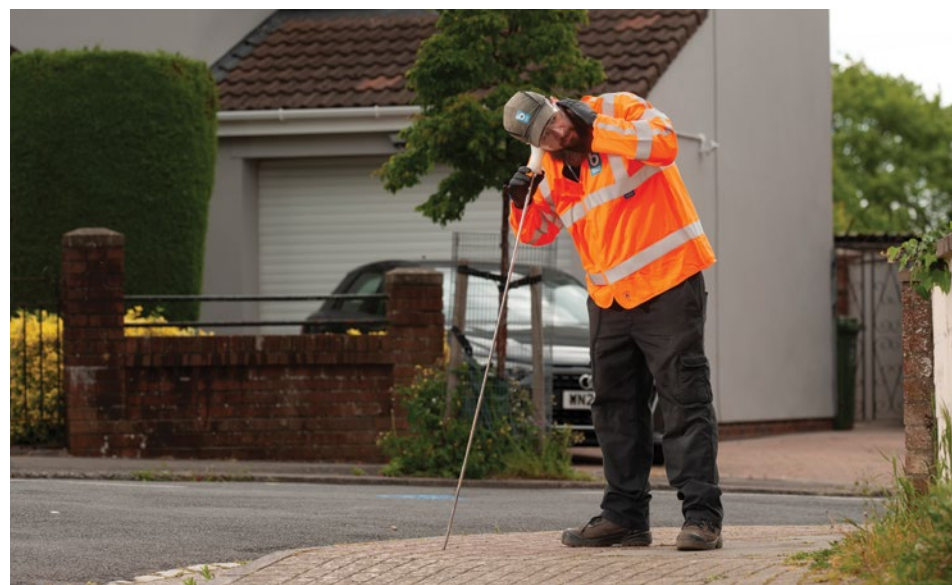
🔍 Leakage detection in Bristol
