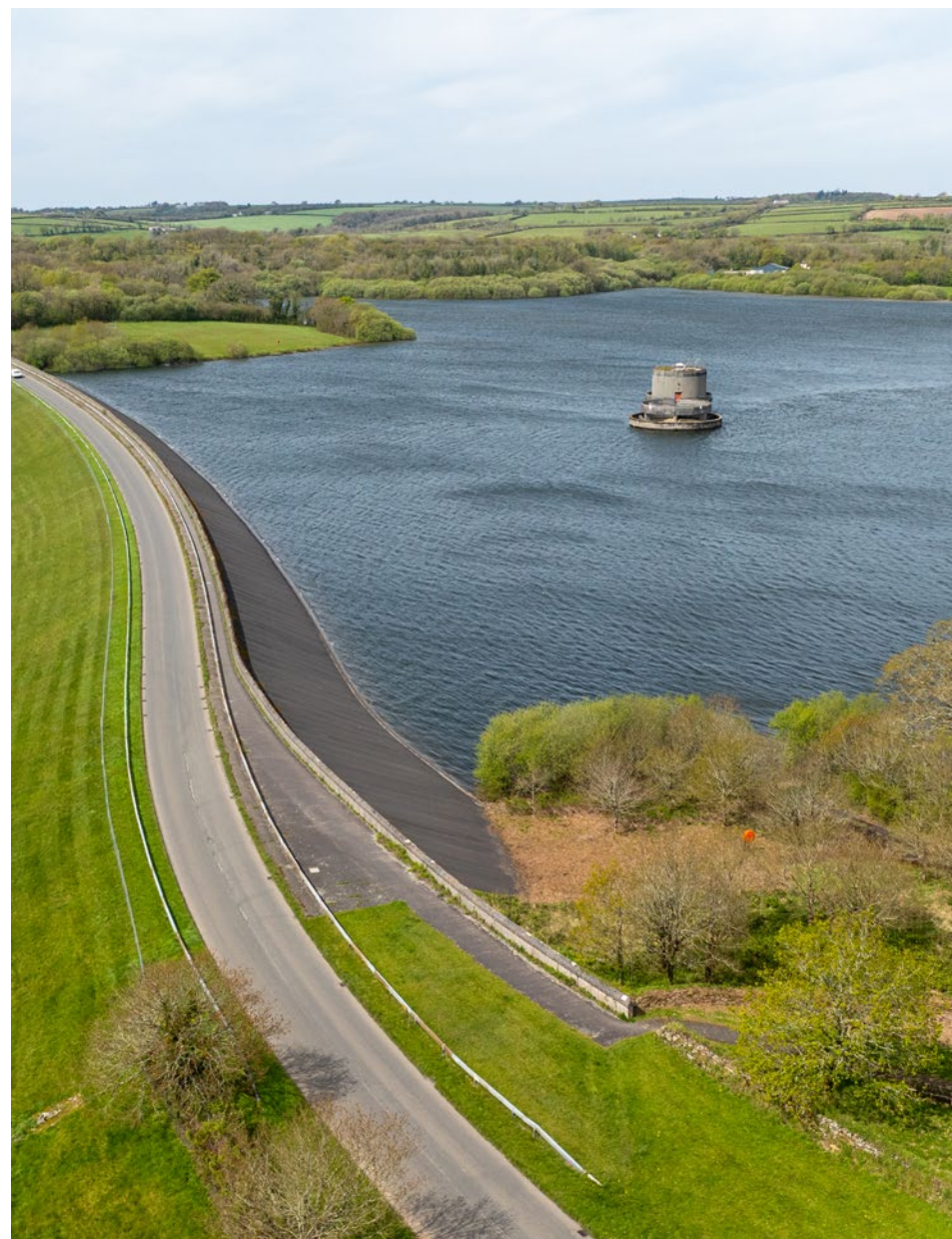
① Roadford reservoir
